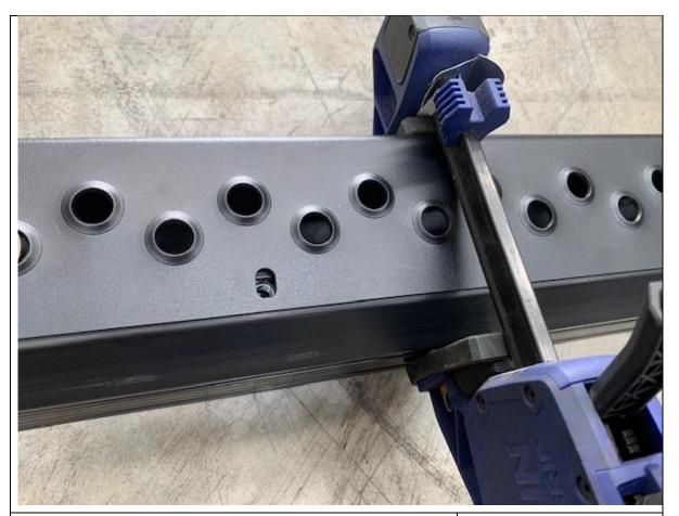
30. Using long tool feed nuts in to centre first and thread in with black M8 button head cap screws and washers
