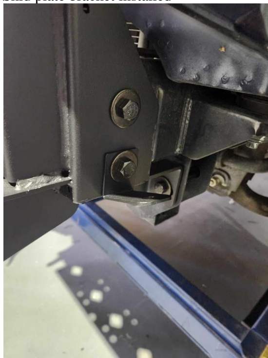
Skid plate bracket installed
